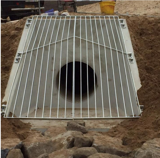
Figure 13: Good examples of culvert grilles (a) at entry; (b) at exit
