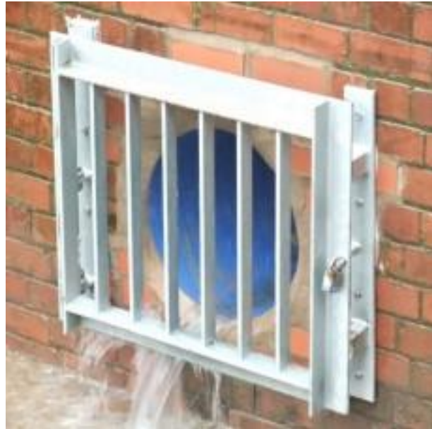
Figure 13: Good examples of culvert grilles (a) at entry; (b) at exit
