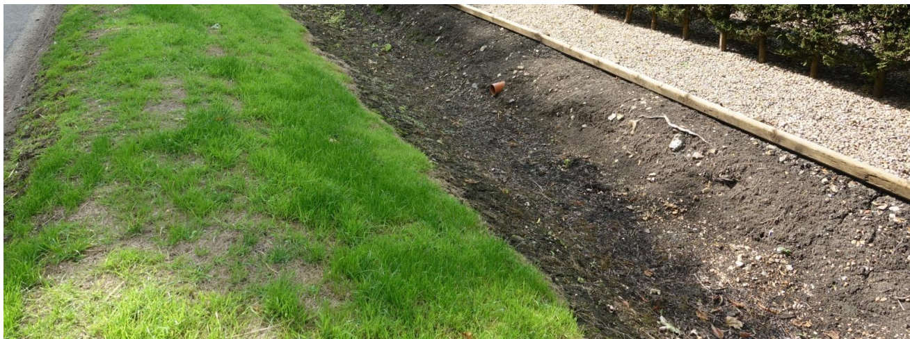
Figure 12: Example of a well-maintained ditch
