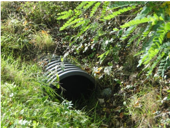
Figure 14: Poor examples of culverts (a) likely to be too small and lacks a grille; (b) grille blocked
