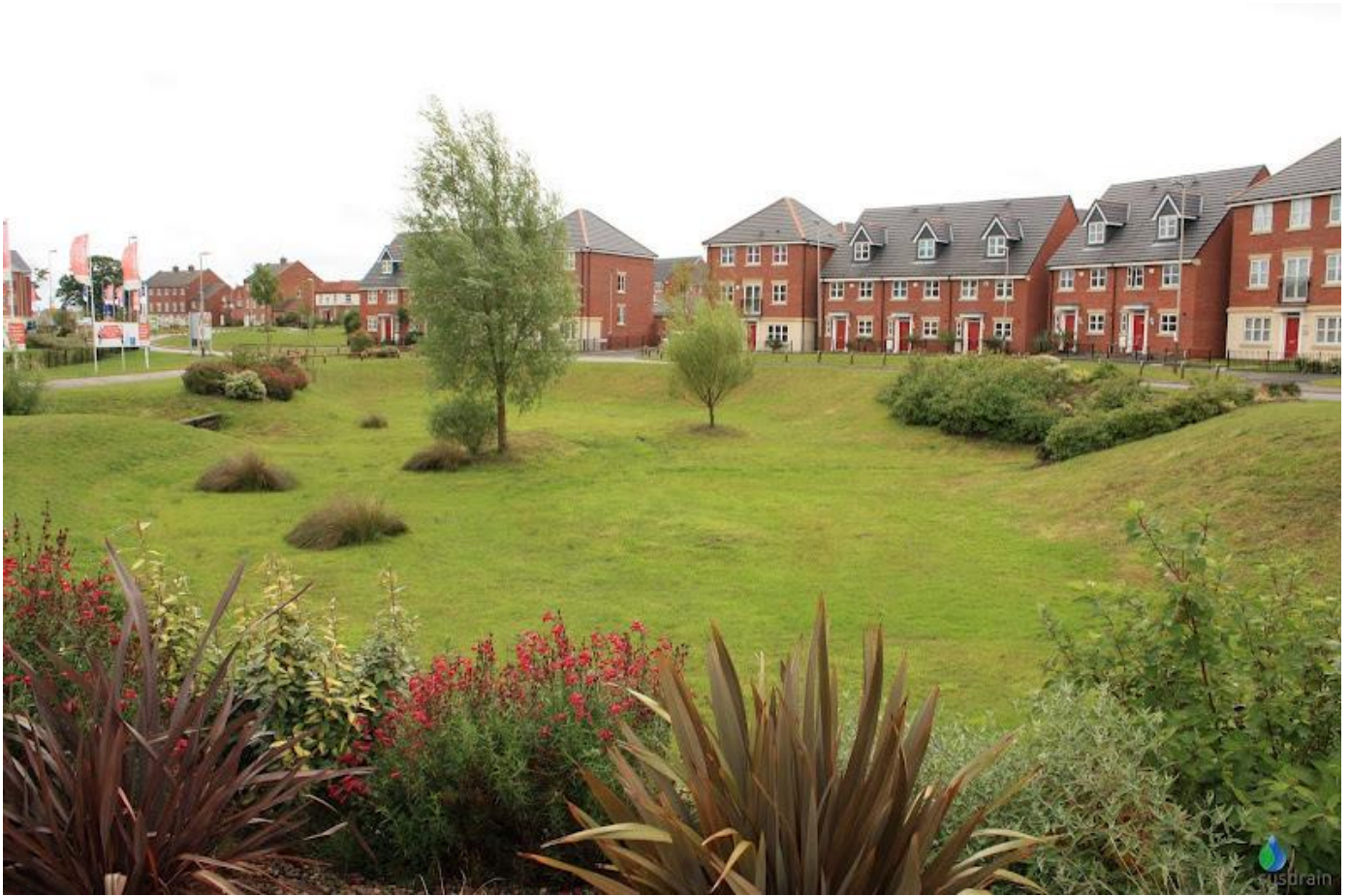
Figure 32: An attenuation basin in a dry condition
