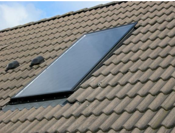
Fig. 33: Roof light and window box solar heat collectors
