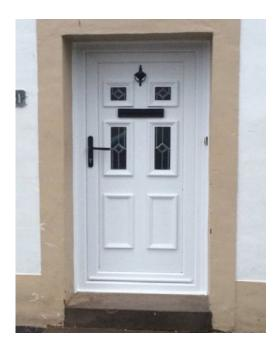
**Figure 5** A flood-resistant door has been installed, which allows additional time for moving items before the water has to be let in. Installation by Floodsafe Projects Ltd (www.floodsafeprojects.co.uk)
