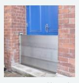
**Figure 2** Demountable type barrier on external door 2 donated by www.lakesidefloodsolutions.co.uk
