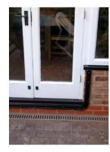
**Figure 1** Non-standard doorway with unobtrusive barrier fittings
