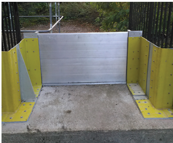
Figure A5.5 Deployment of a floodgate defence system to prevent water entering the site (courtesy Adler & Allen)
