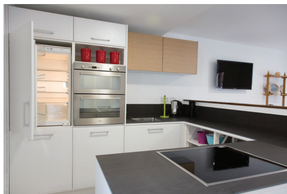
Figure 24.3 Flood recoverable kitchen. This kitchen, installed as part of the BRE flood-resilient repair house, showcases raised electrical appliances and sockets, as well as composite materials for cupboard doors and a stonework finish on the worktops (courtesy BRE)
