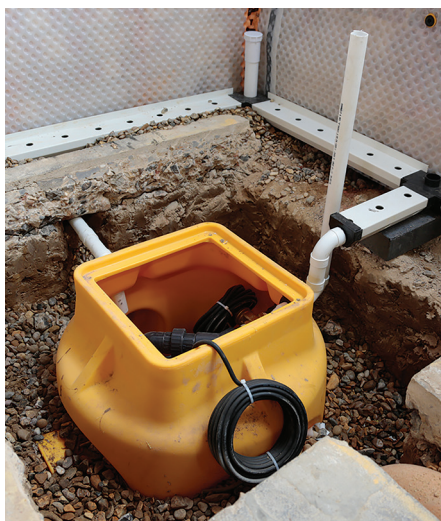
Figure 24.1 Example of a sump and pump system (courtesy Peter White, BRE)
