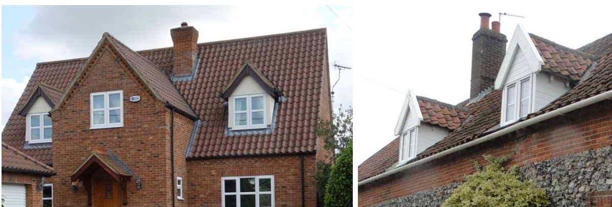
Fig. 15: Various dormer windows
