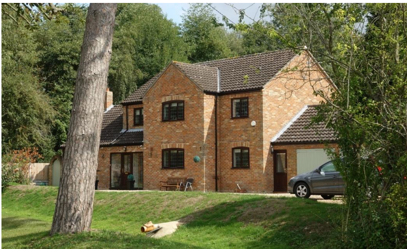
Fig. 8: 20th century buff brick house
