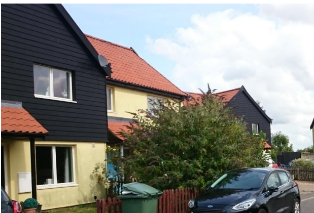
Fig. 12: Inappropriate use of timber cladding
