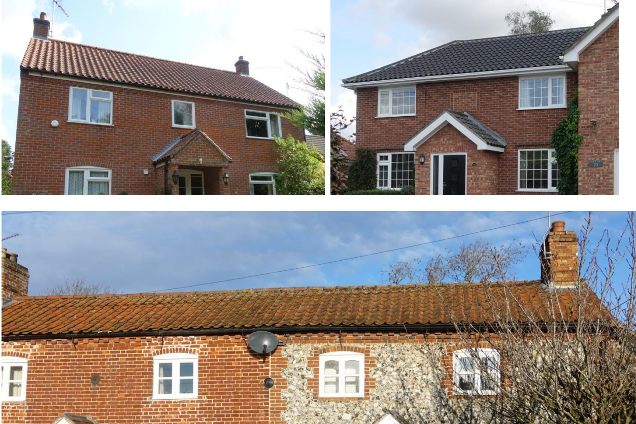
Fig. 13: Various pantile roofs
